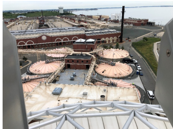
Gravity Thickeners 1 through 6
