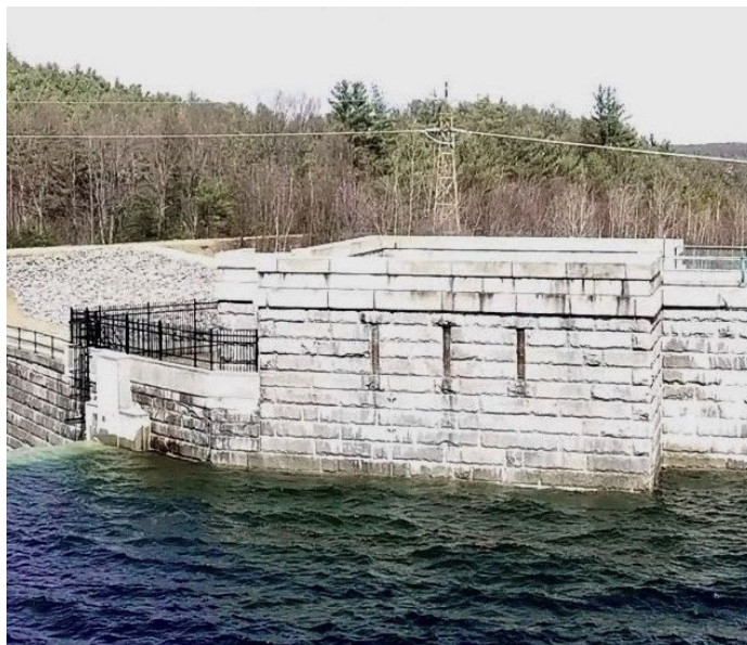
Exterior of Bastion
