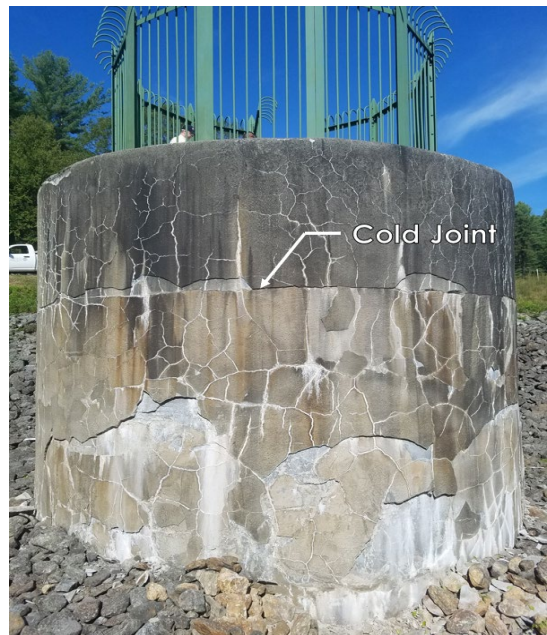
Shaft 2 Preconstruction Condition
