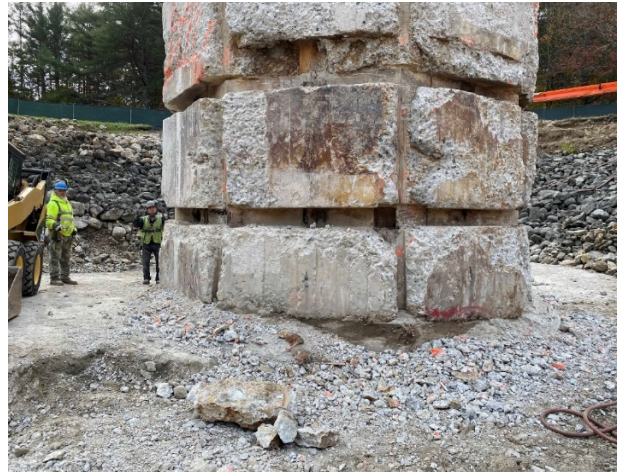
Horizontal and vertical timbers and concrete panels removed
